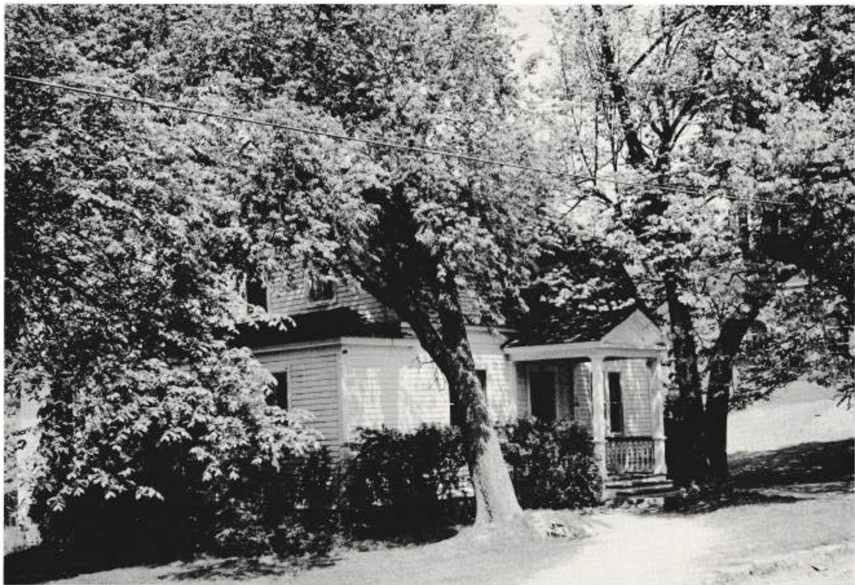
The Clubhouse located on the upper end of the intra-mural is the gathering place of the college. The modern lunch room, barber shop, and lounge make a contribution of fellowship and friendliness.
