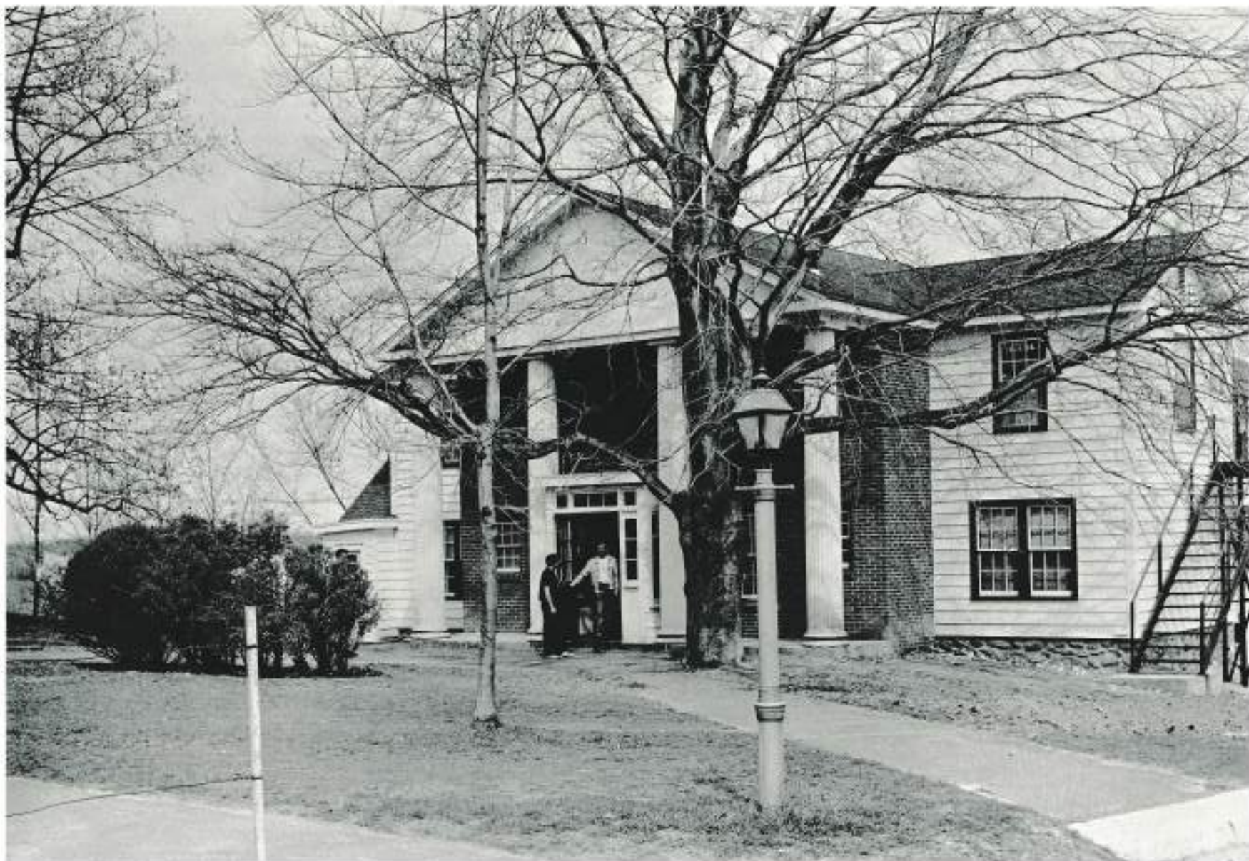
T-Hall, one of the smaller dormitories on the campus, has recently been completely renovated. It overlooks the new athletic fields and college golf course.
